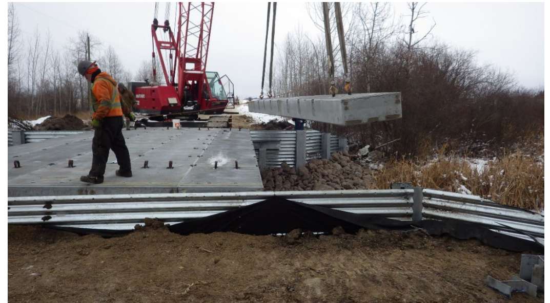
BF72902 - Twp 614 Bridge, east of RR 485
