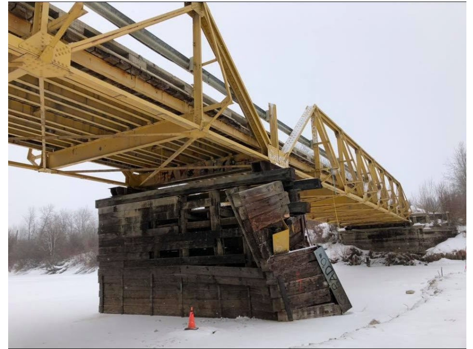
BF9595 - Lessard Road Bridge over Beaver River
