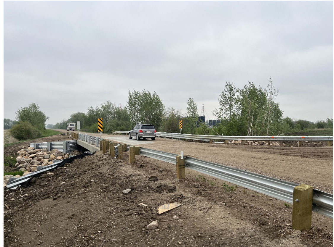
BF72746 - RR 434 Bridge, south of Hwy 28
