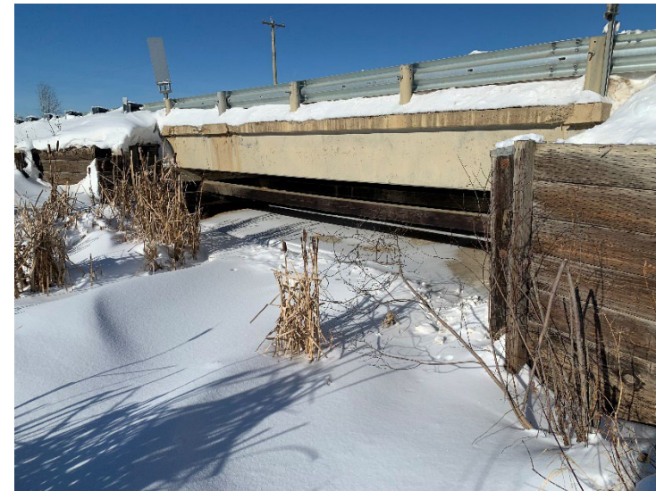
BF72115 - Twp 640 Bridge, east of RR 473
