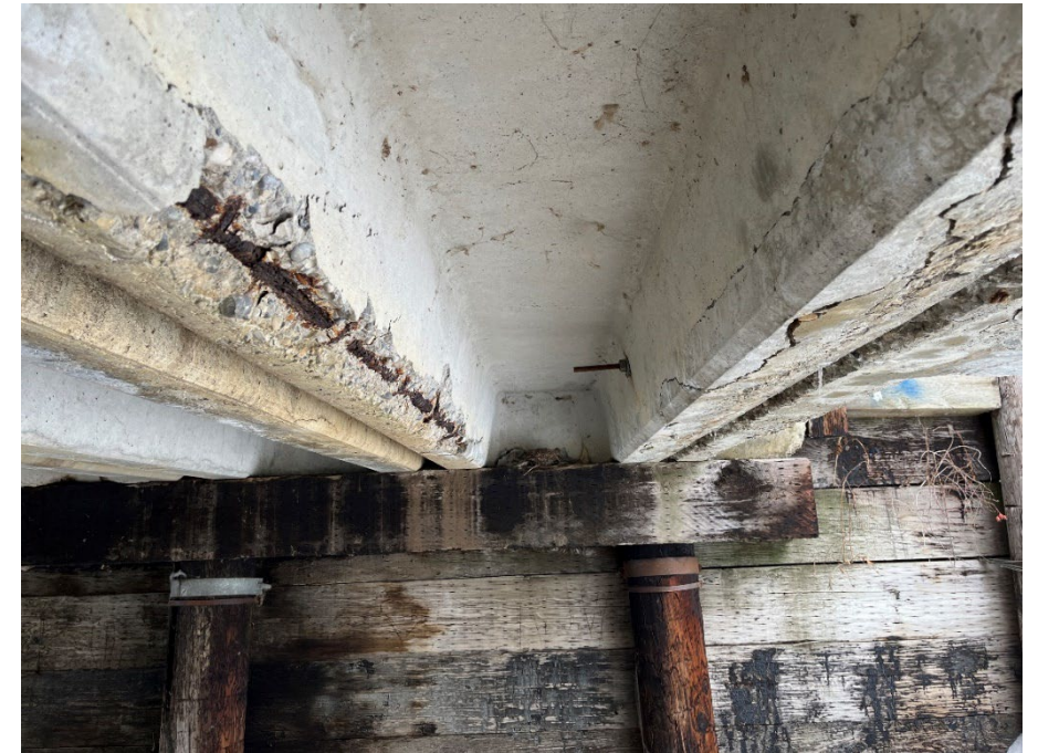
BF78069 - Twp Rd 615 (50 Ave) Bridge, east of Fort Kent
