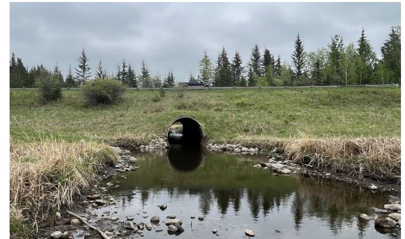
BF78682 – Twp 634 Bridge Culvert, west of RR 424
