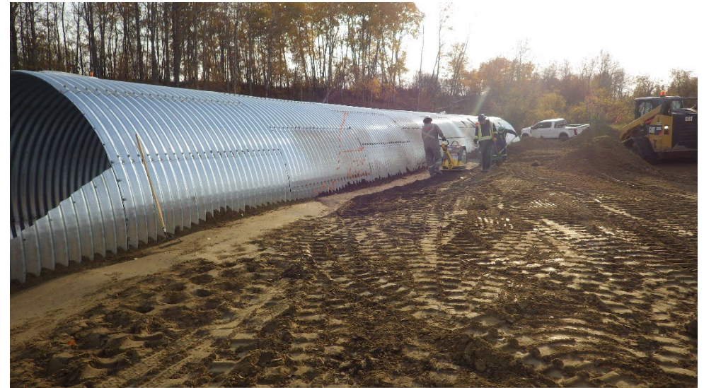
BF73660 - RR 485 Bridge Culvert, south of Hwy 28
