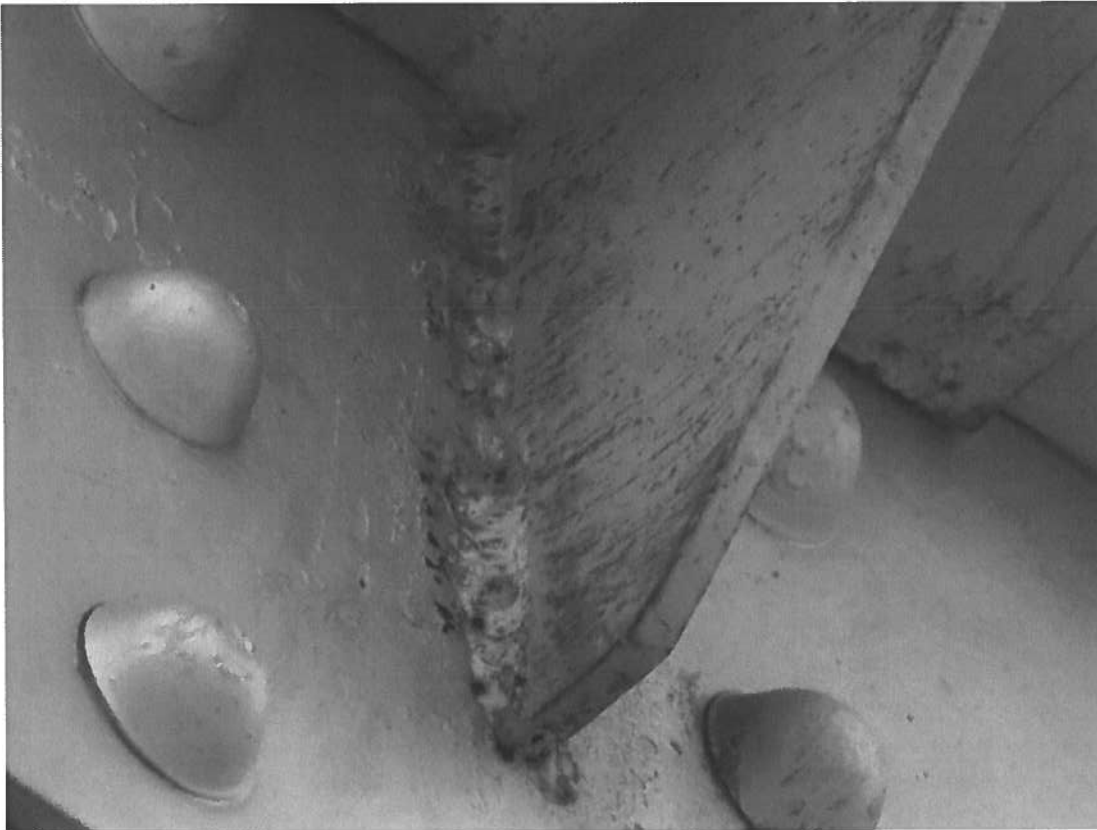
U8U8W welded connection, south view
