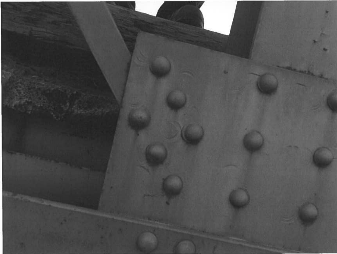
U2L3 bottom connection exterior
