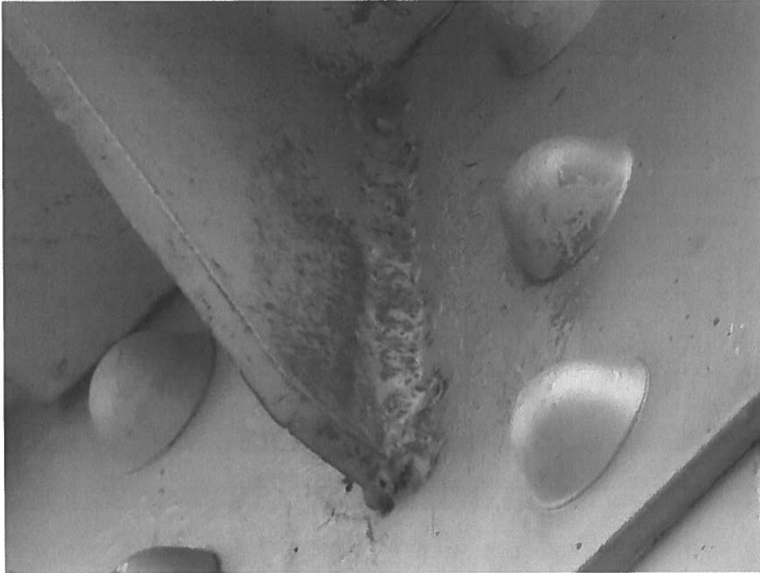
U8U8W welded connection-north view
