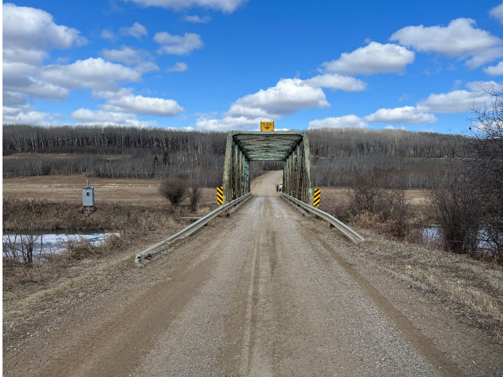
BF72355 – Range Road 410 over Beaver River – “Aylesworth” Bridge
