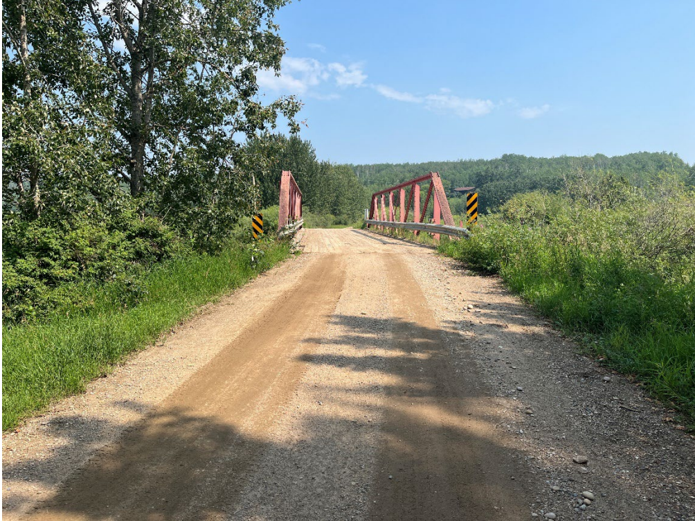
BF7431 – Township Road 624 over Beaver River – “Tillers” Bridge
