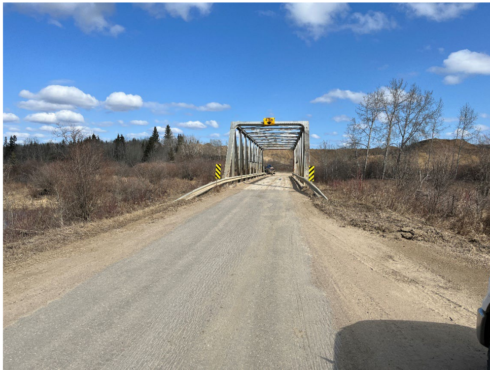
BF72515 – Range Road 485A over Beaver River – “Truman” Bridge
