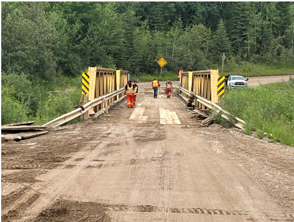
BF9595 – Range Road 452A over Beaver River – “Lessard” Bridge
